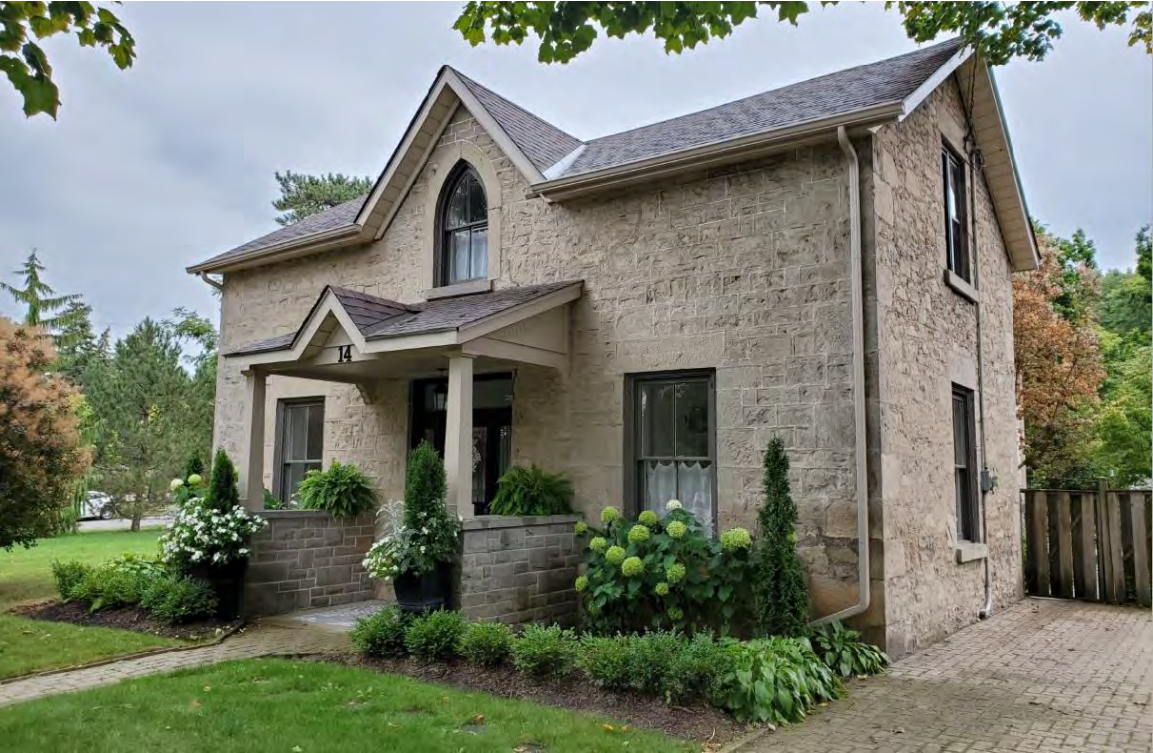
Current photos of the subject site (14 Forbes Avenue)
