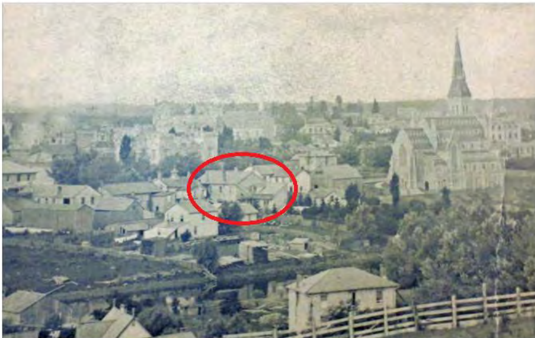
from Grange Street looking towards Woolwich Street (69 Woolwich in the centre with 1½ storey rear addition) 1875
